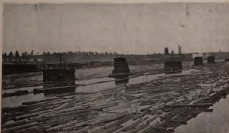
FIG. 108. — Piers built in a River to hold Storage Booms in Place. Minnesota.
